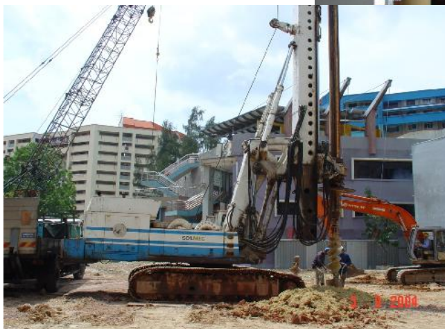
bored piles for building extension
