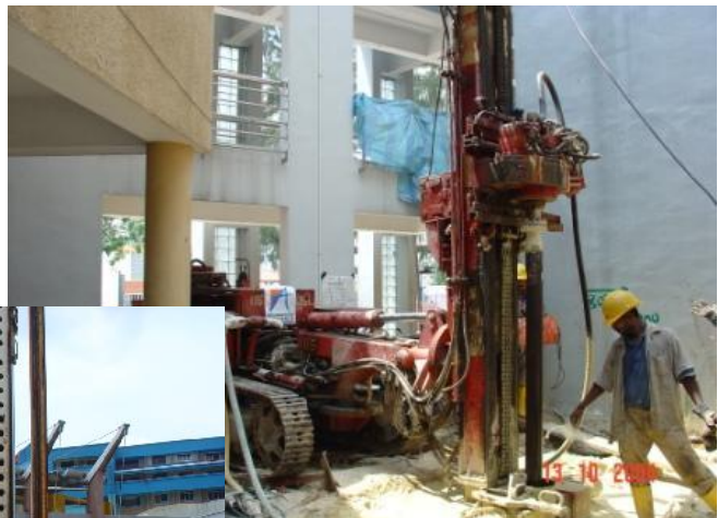
micropiles for new lift
