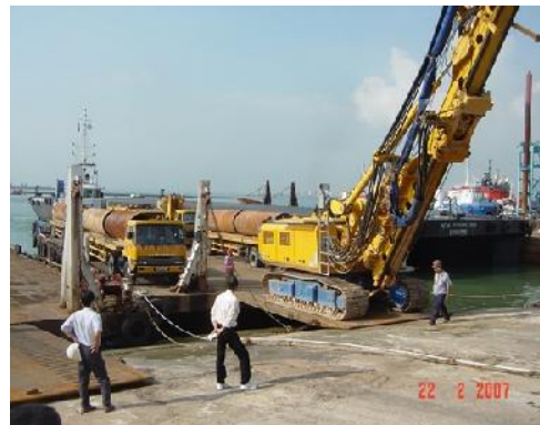
loading boring rig & casings on barge for Pulau Ular
