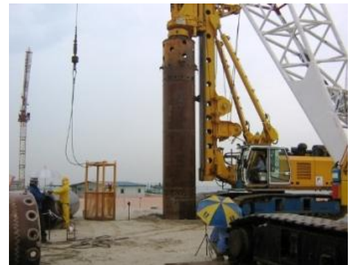
Bauer BG28 installing double wall casing
