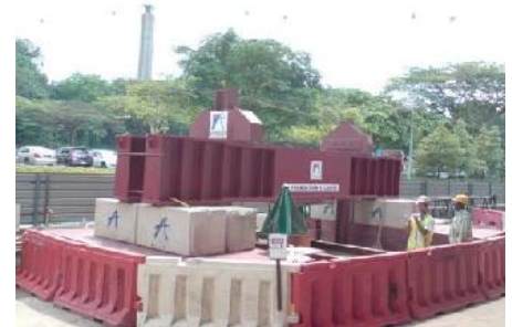
Test pile by Reaction Tension Piles
