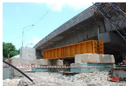
Pile load test by tension reaction piles
