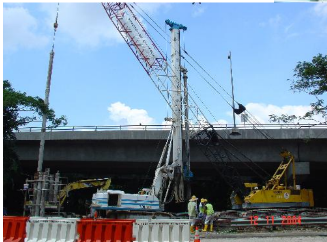
Foundation bored pile installation
