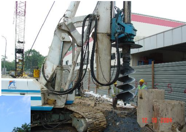
Contiguous bored pile installation
