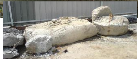
slab / wall reinforced concrete cored by boring rig
