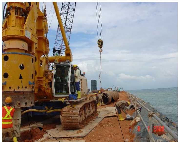
guide wall double wall casing rotary drive turn table for casing installation
